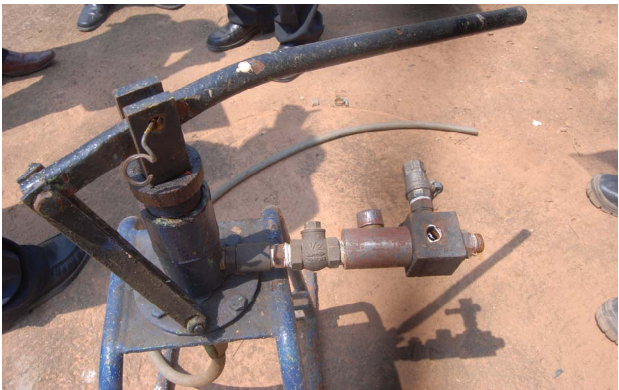
Photo 7: The hydrotest set up does not have relief valve.
